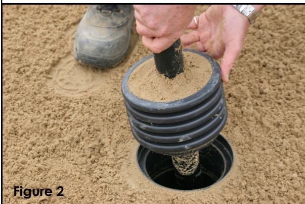
Figure 2. Remove both together, keeping sand trapped in the maintenance pipe.
