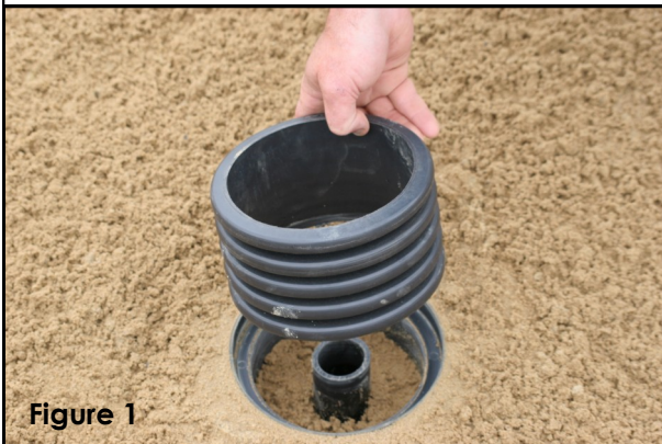
Figure 1. Remove grill. Place maintenance pipe onto top of unit and pull plunger up until the disc is level with the bottom of the maintenance pipe.
