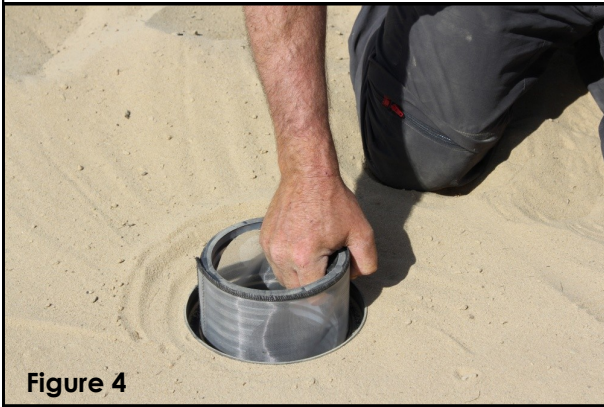
Figure 4. Carefully insert bucket (with screen attached) into unit ensuring holes in bucket line up with drainage pipe.
